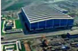
L&T-MHPS Turbine Generators
