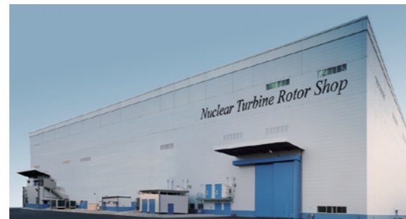
Nuclear Turbine Shop
