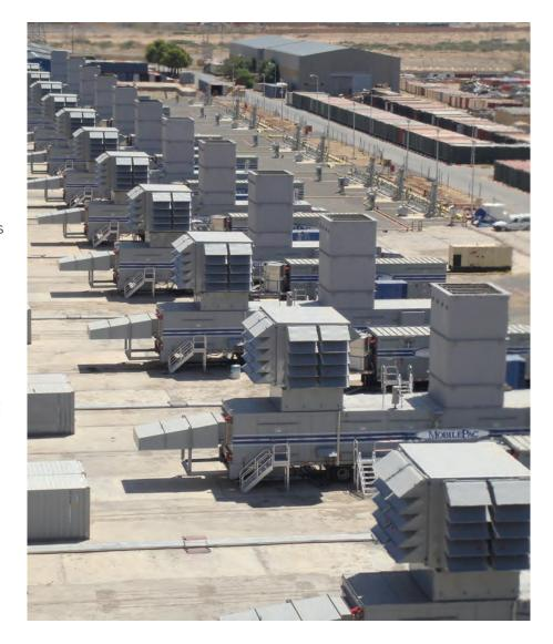
Multiple MOBILEPAC® units can be deployed for data center applications. Mitsubishi Power Aero can offer balance of plant, EPC services, full turnkey installation, and interconnection to the grid or a standalone microgrid with load sharing capability.
