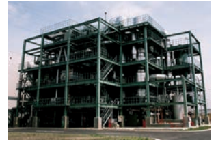
汚泥焼却施設 Sludge incineration facility
