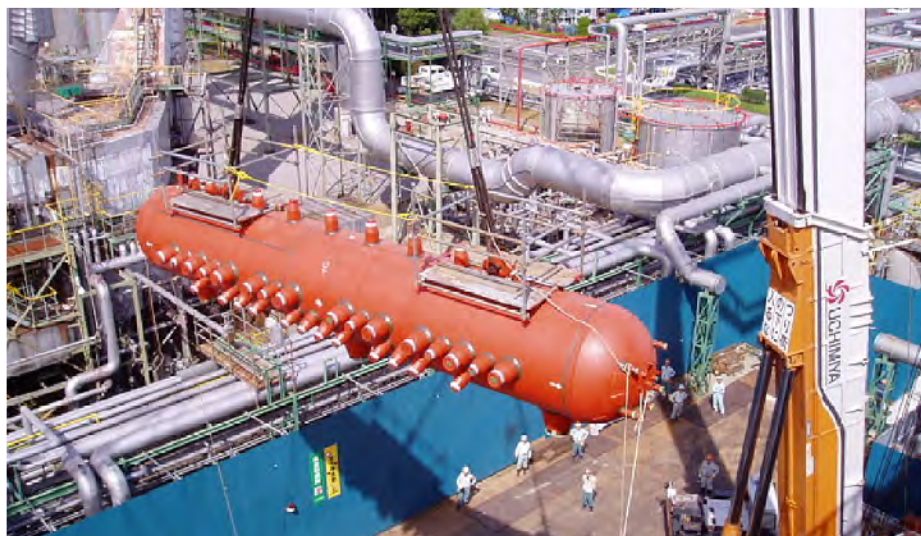
265t/h 単胴水管型自家発電用ボイラ据付 Installation of 265t/h one drum water tube boiler for self power generation
