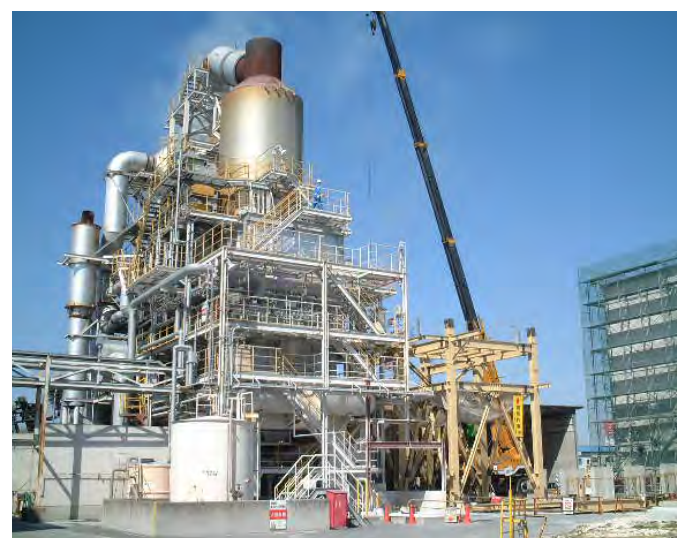
焼却炉用排熱ボイラ据付 Installation of exhaust heat recovery boiler for incinerator
