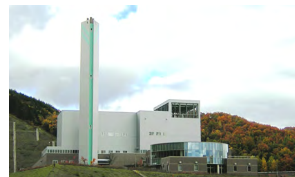
55t/24h×3炉 発電付流動床式焼却施設 Fluidized-bed type incinerator with generating equipment (55t/24h×3 incinerators)
