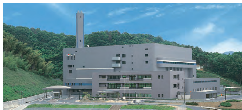
110t/24h×3炉 発電付流動床式焼却施設 Fluidized-bed type incinerator with generating equipment (110t/24h×3 incinerators)
