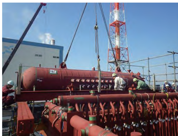
耐圧部据付（ドラム、水壁管上部） Installation of pressure part (drum, upper part of water wall)
