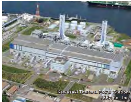
Gas Turbine Combined Cycle (GTCC) Power Plant
