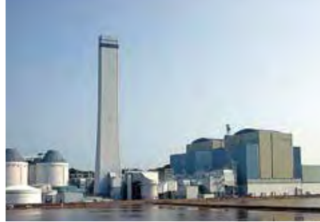
1,050 MW Coal-Fired Once-Through Boiler
