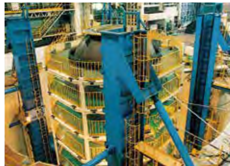
Pressure Vessel Hydrostatic Test Pit
