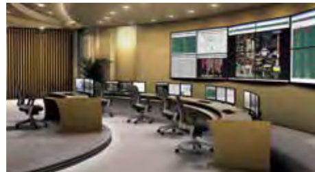
Plant Control System
