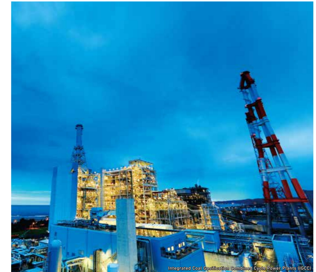
Integrated Coal Gasification Combined Cycle Power Plants (IGCC)
