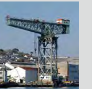
Giant Cantilever Crane (Not open to public)
