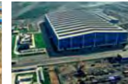
L&T-MHI Power Turbine Generators
