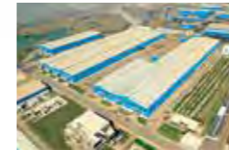
L&T-MHI Power Boilers
