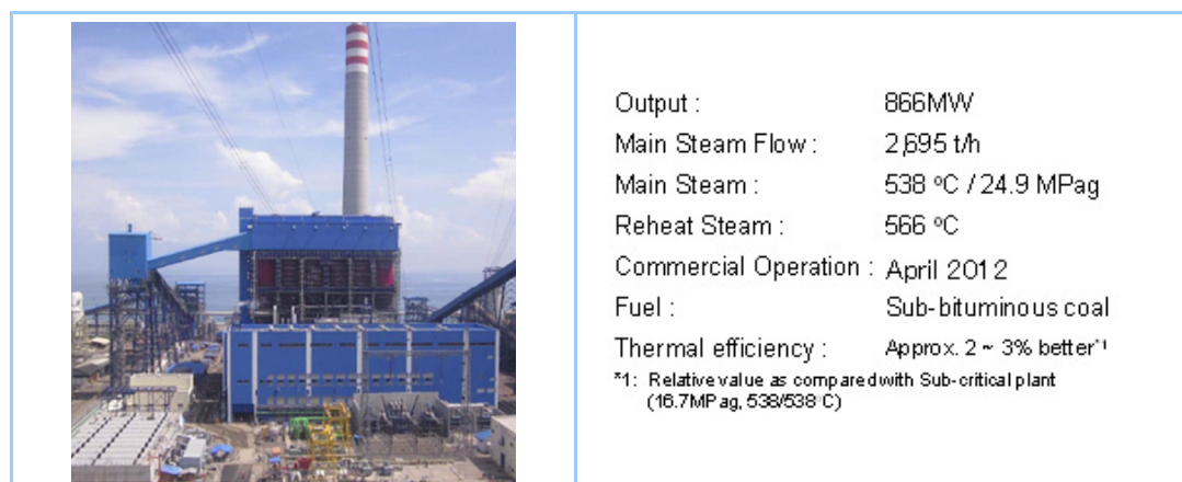
Figure 4 Subbituminous coal-fired SC boiler, Paiton II (Indonesia)
