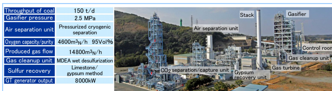
Figure 7 Pilot plant outline for the research and development of coal gasification technology with innovative CO 2 capture (Coal Energy Application for Gas, Liquid and Electricity: EAGLE-STEP 3)
