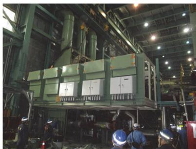
**Figure 4 Installation of new fuel gas unit**
