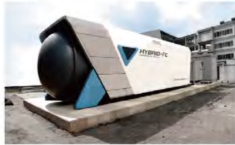
Figure 8 SOFC-MGT hybrid system for demonstration delivered to Kyushu University
