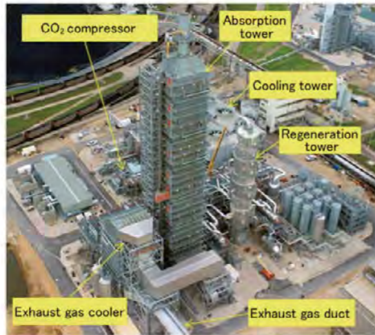
NRG Energy, Inc. and JX Nippon Oil & Gas Exploration Corporation Photo of Petra Nova project
