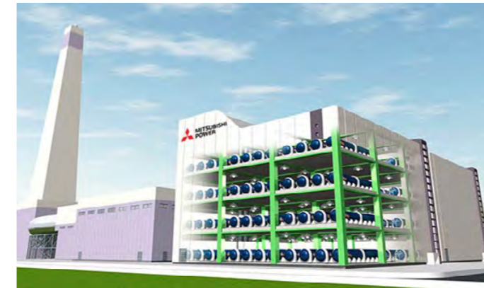
Figure 1: Gas Turbine Fuel Cell combined-cycle Power Plant
