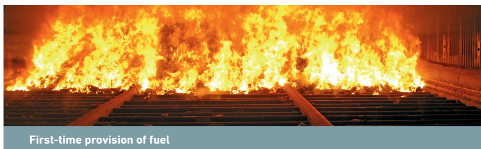
3-track stoker firing grate during installation
