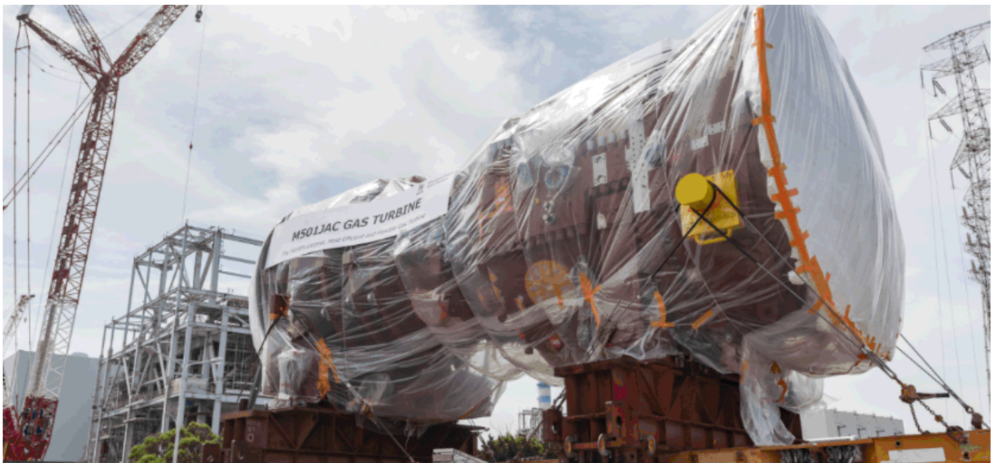
Transporting the M501JAC to T-Point 2.
