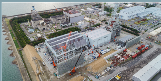
T-Point 2 during construction, October 2019.
