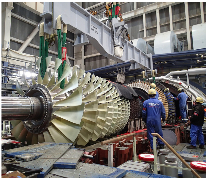
M501JAC rotor installation.
